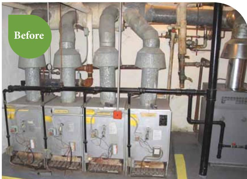
*Before: Pre-existing condition of the five boilers which generate heat and hot water to the buildings located at 152-164 Manhattan Ave. at 107th Street.*
