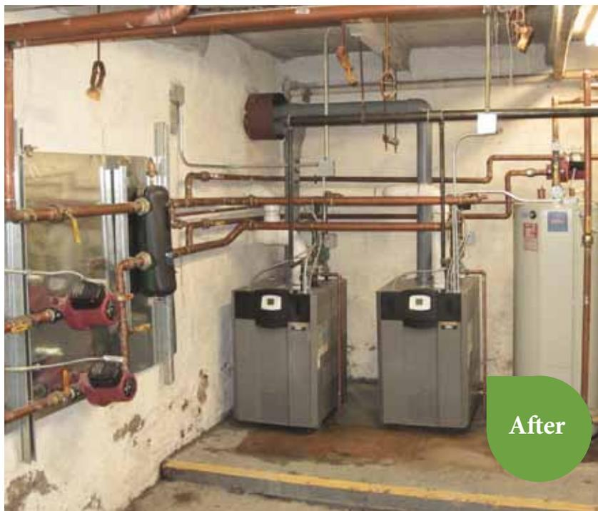
*After: Thanks to HCC's Weatherization Assistance Program, we replaced the entire five boilers and installed two energy-efficient boilers.*
